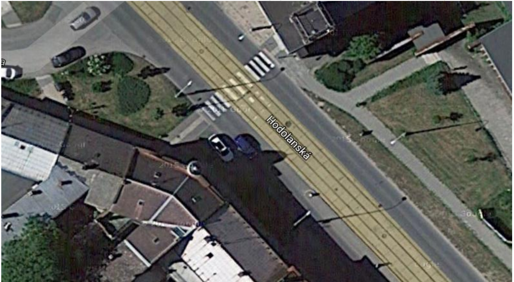
Hodolanska street, non-standardised pedestrian crossing before removal
